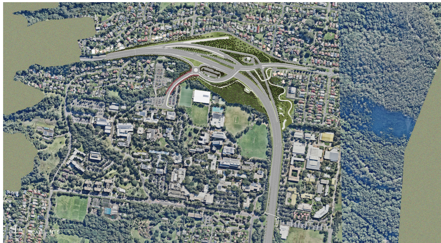
Figure 4: Mount Ousley interchange, the Project
